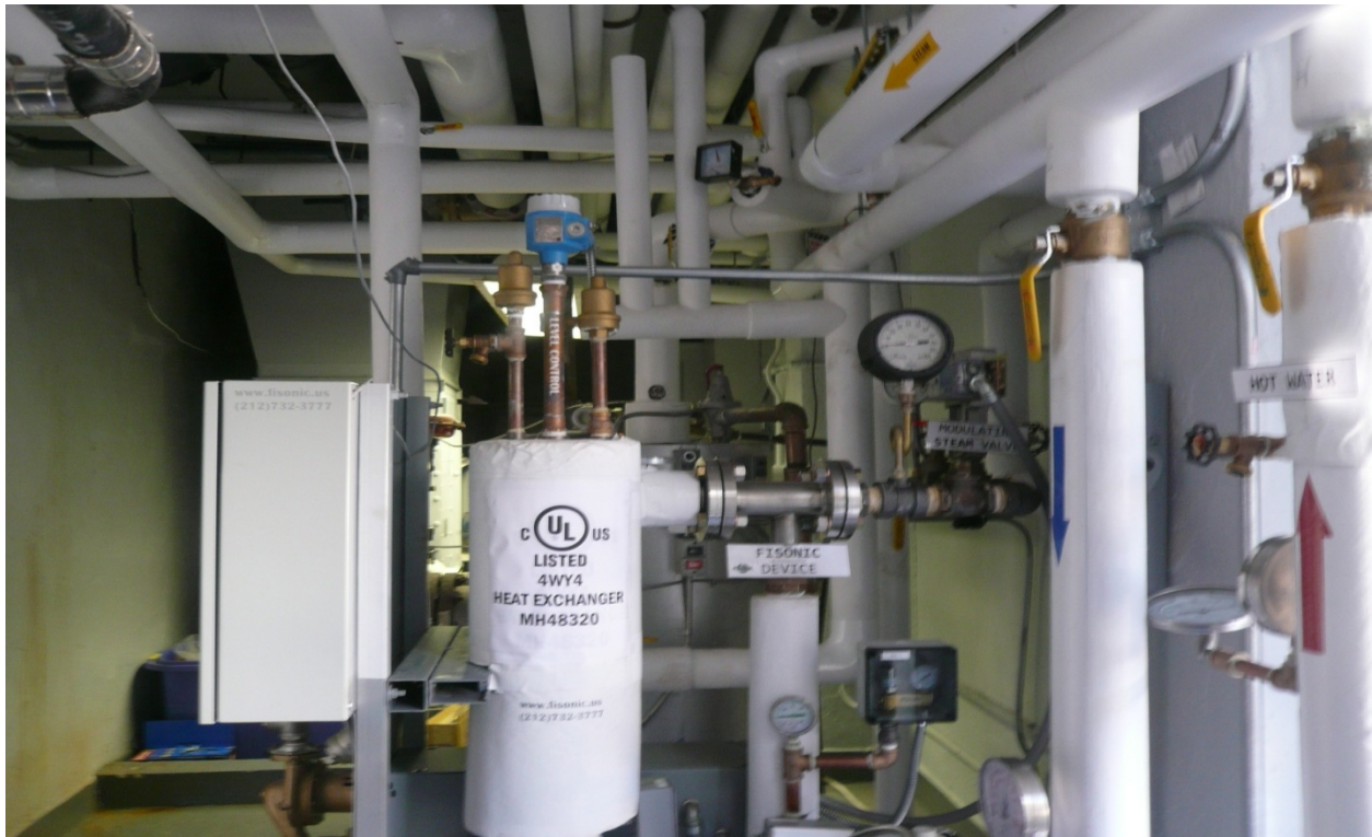
Figure 40. New Domestic Hot Water Unit with the Fisonic Pumping Device
